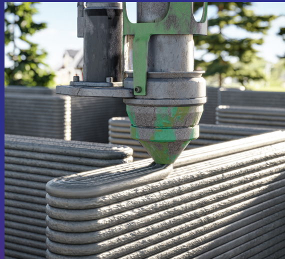
Figure 5: 3D printed cement walls
