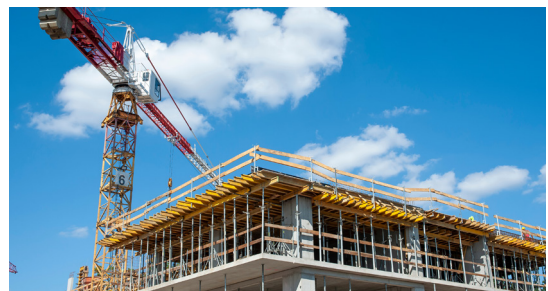
Figure 2: A building under construction.
