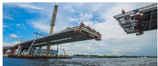
Figure 3: A bridge under construction.
