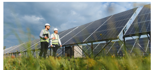
Figure 1: Solar panels, used to convert energy from sunlight.
