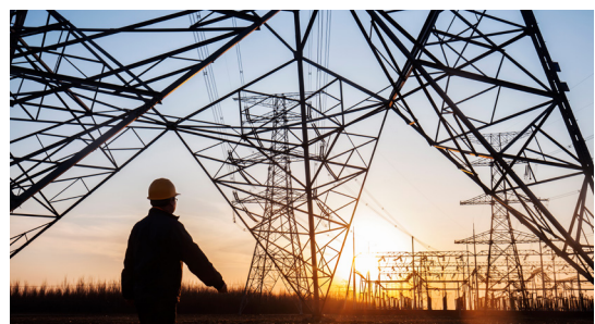
Figure 2: A photo of electricity pylons carrying high-voltage electricity.
