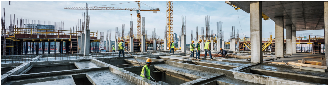
Figure 5: Construction workers assemble a skyscraper's steel framework, creating the structure that supports the building's weight and resists wind forces.
