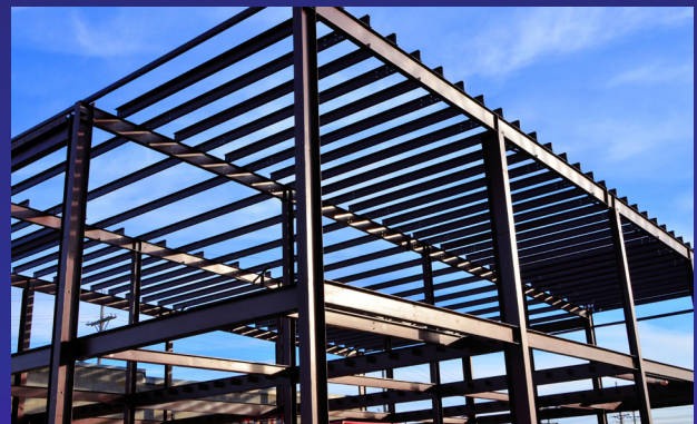
Figure 4: Unlike wood framing, a steel structure provides greater strength and allows commercial buildings to span larger spaces with fewer supports.
